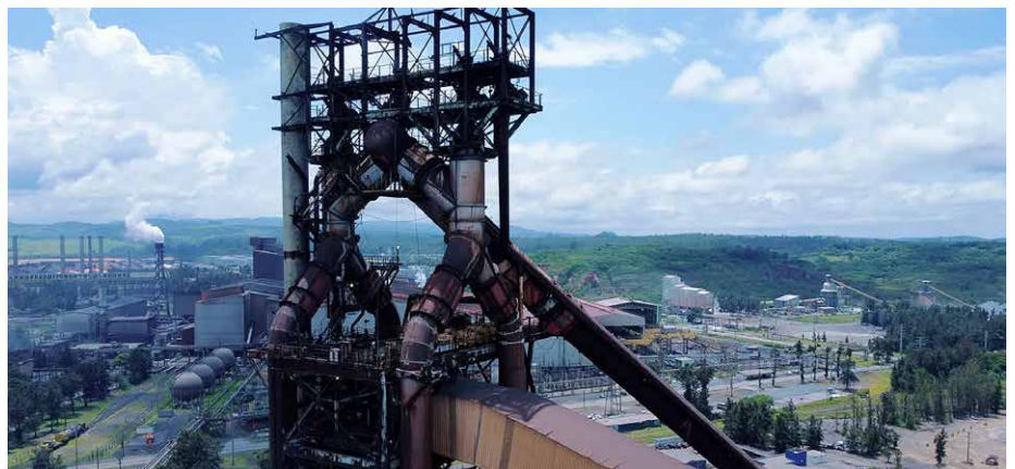
Gerdau plans a major upgrade of its blast furnace (Photo: Danieli Corus)
