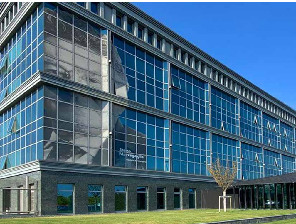
Headquarters of Marcegaglia Group in Gazoldo degli Ippoliti, Mantova, Italy (Picture: Marcegaglia)
