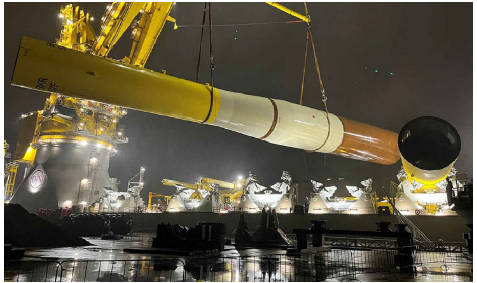
Shipment of monopile foundations for offshore wind turbines (Picture: Ørsted)
