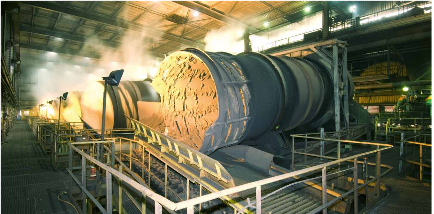
Pelletising plant at Tata Steel's IJmuiden works (Picture from the archives © Tata Steel Europe)
