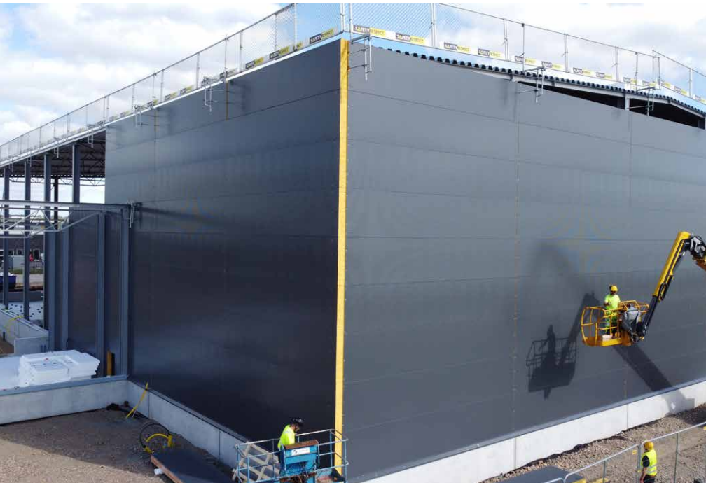
Fossil-free steel has been used for the sandwich panels (Picture: Anna Malm)
