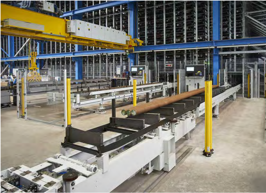
The storage system can feed the adjacent sawing centre with material via special saw cassettes and automatically longitudinal moving carriages (Picture: Kasto)
