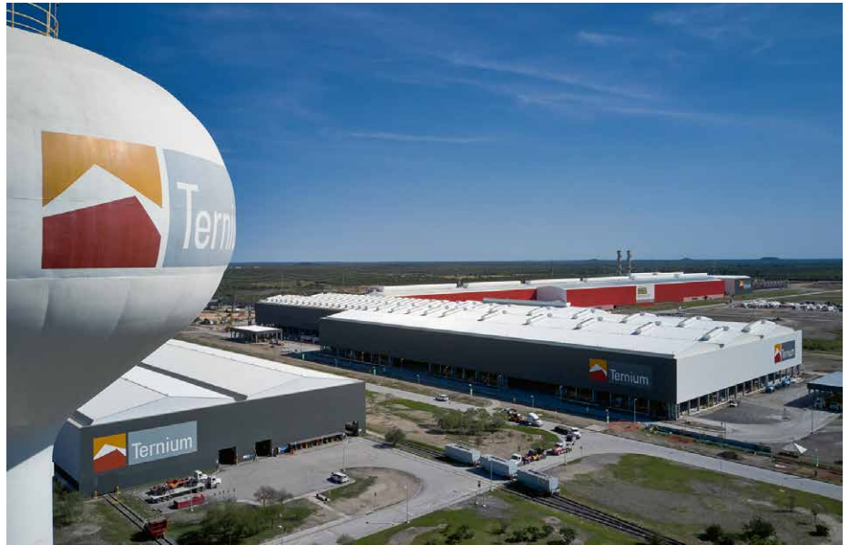
The new steel plant will integrate Ternium's downstream operations in Pesquería
