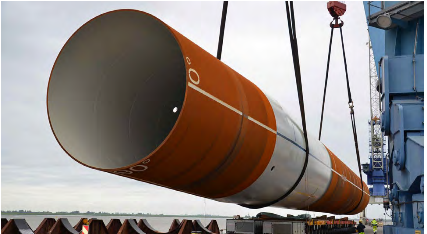
Loading out of a monopile foundation at the operation terminal (Archive picture: Steelwind Nordenham)
