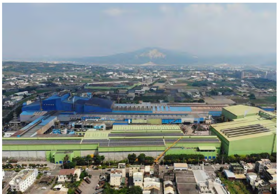
Feng Hsin Steel operates a mini-mill with an annual capacity of 2 million t of rebar, structural steel and SBQ products (Picture: BSE)
