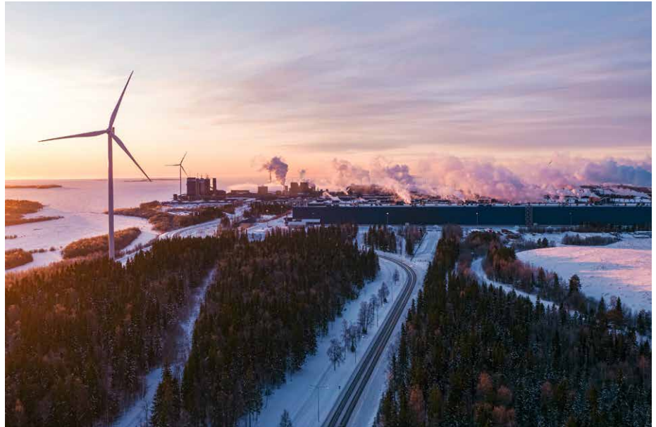
Outokumpu's largest steelmaking mill is situated in Tornio, Finland (Photo: Outokumpu)
