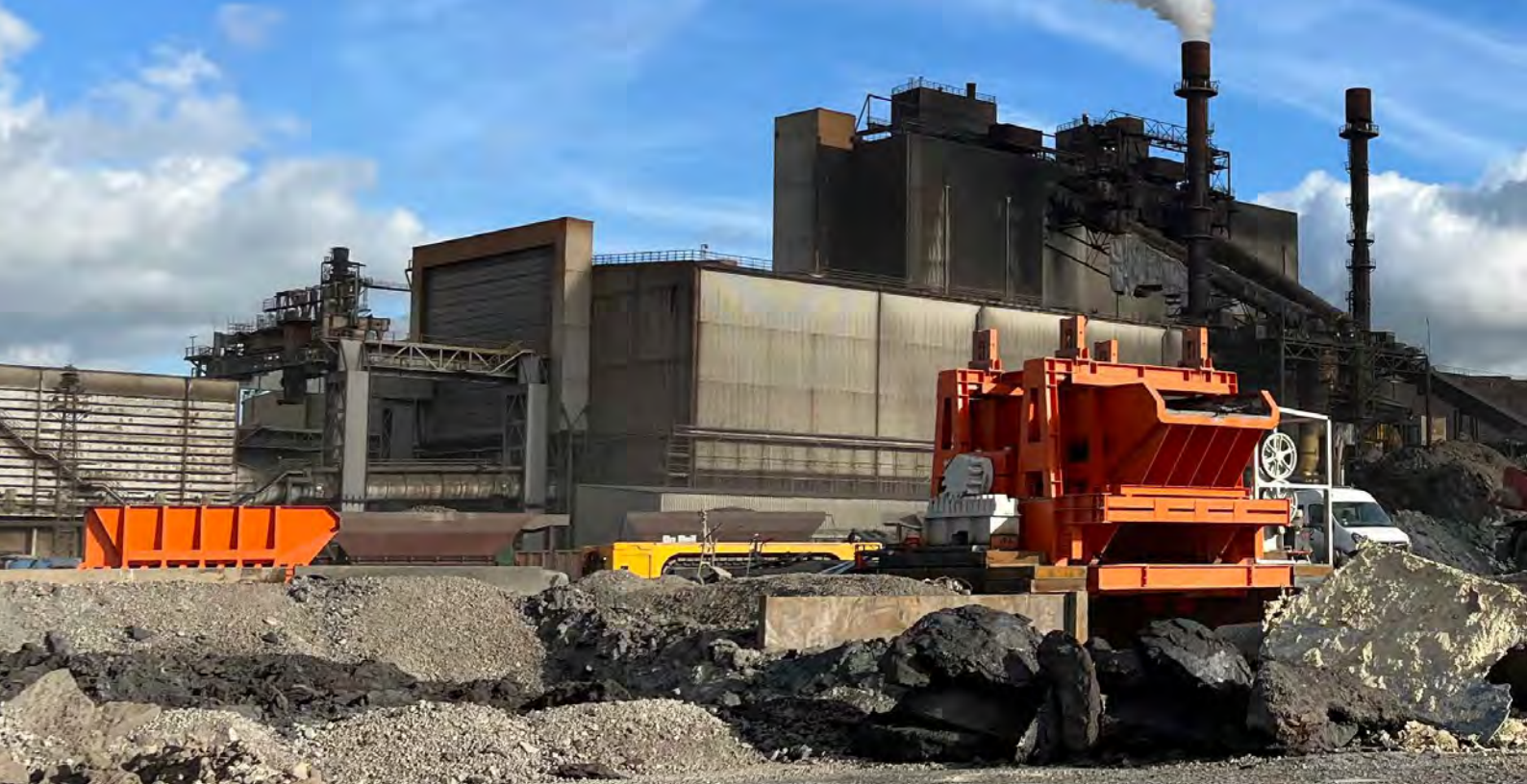
Hot Box Mover, Hot Box and the tipping device in the outside area of the steel plant (Picture: TML)
