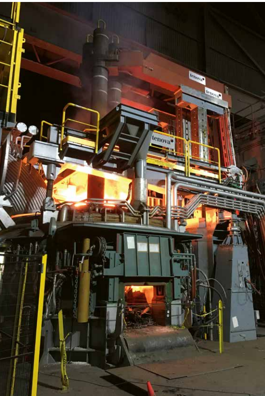
Valbruna ASW has successfully commissioned its newly installed EAF (Photo: Tenova)
