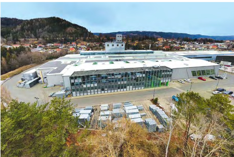
Judenburg works is one of five production sites within the Wuppermann Group (Picture: Wuppermann)
