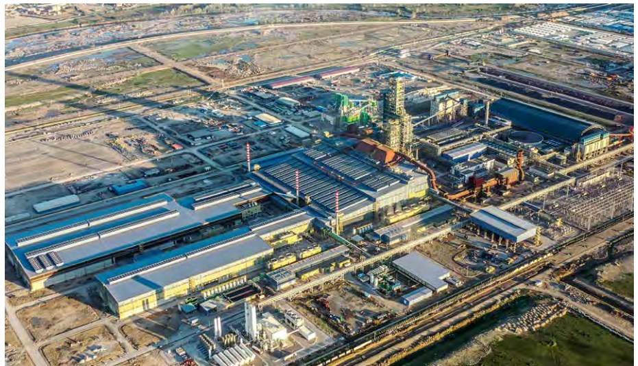
The DRI plant of Algerian Qatari Steel (AQS) was supplied by Midrex and Paul Wurth as consortium partners (Picture: SMS group)
