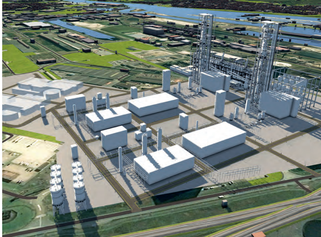
This computer graphic already shows a later expansion stage with two DRI-REF production units (Picture: Tata Steel)
