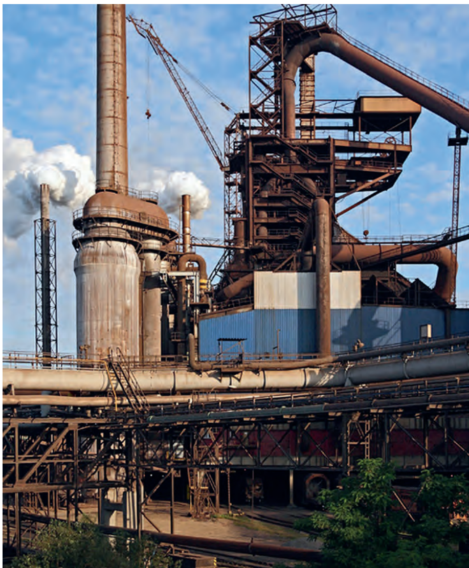
At Trinec Iron and Steel Works a hot blast stove at blast furnace No. 4 is to be replaced by a new one (Picture: Trinecké Železářny)
