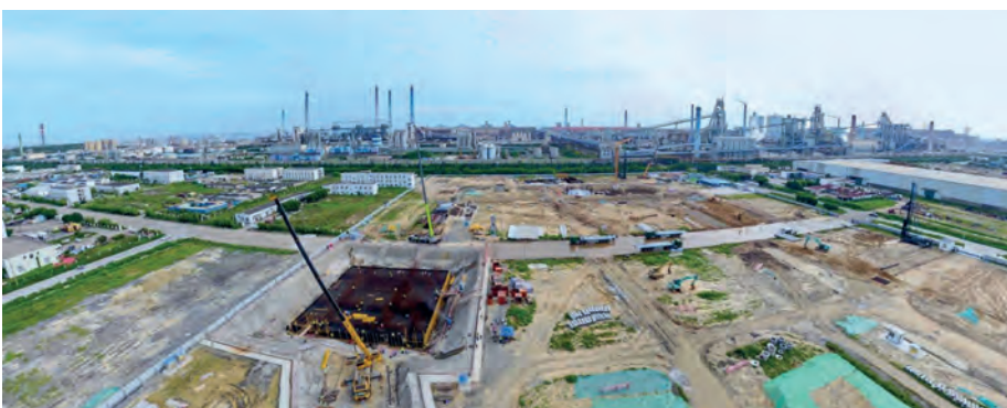
Construction site for new DRI project (Photo: Danieli)
