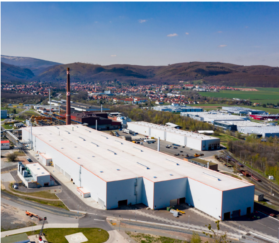
The new heat-treatment facilities at Ilsenburger Grobblech are accommodated in a complex of three new buildings covering an area of 31.290 square metres (Picture: Ilsenburger Grobblech GmbH)
