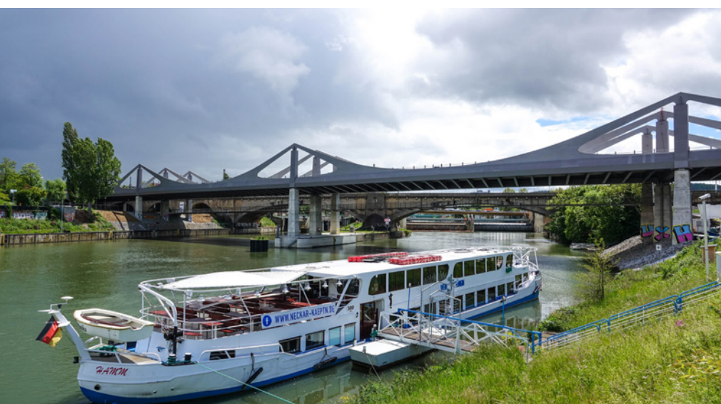
Striking steel sails identify the two main spans above the river (Picture: schlaich bergemann partner/Frank Schächner)
