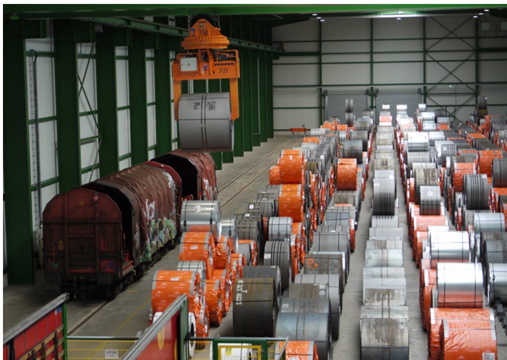
In the new coil logistics facility, TWMS/metals provides maximum automation of train unloading, coil storage and truck loading activities (Picture: 3tn)
