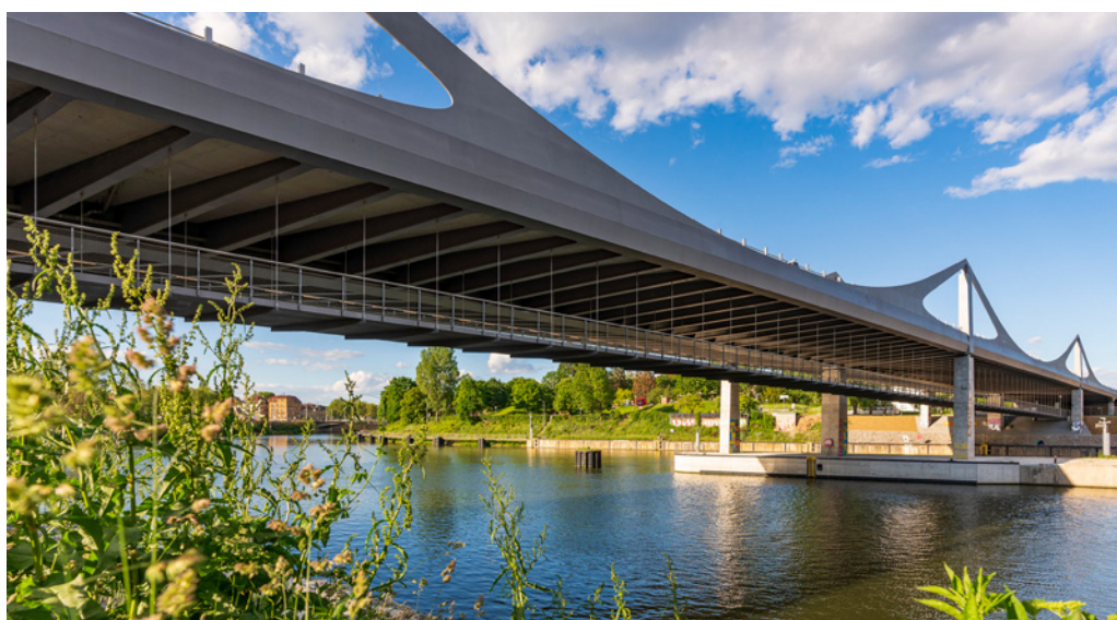
The sbp engineers aimed for a visually lightweight bridge structure, despite the span of nearly 80 metres (Picture: schlaich bergemann partner/Andreas Schnubel)
