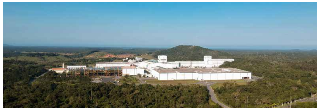
ArcelorMittal Vega's flat rolling complex will undergo comprehensive expansion (Picture: SMS group)
