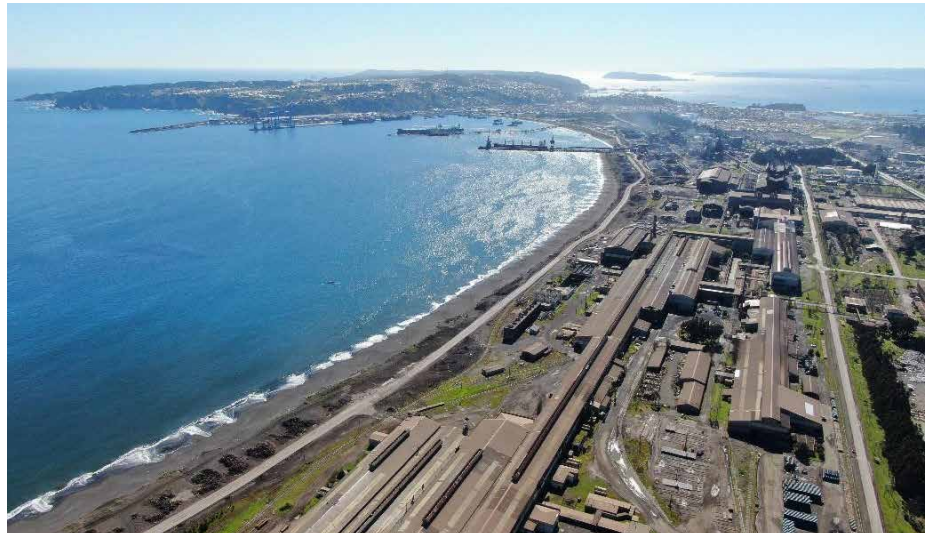
Compañía Siderúrgica Huachipato (CSH) facilities in Chile (Picture: SMS group)
