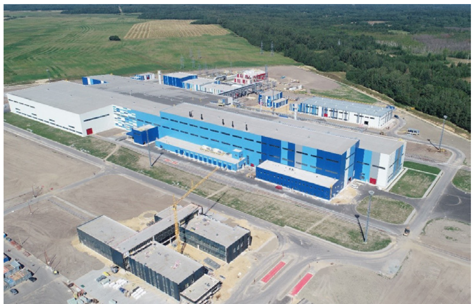
This ultra-modern cold strip production facility has been established for Miory Steel in the north of Belarus (Picture: SMS group)
