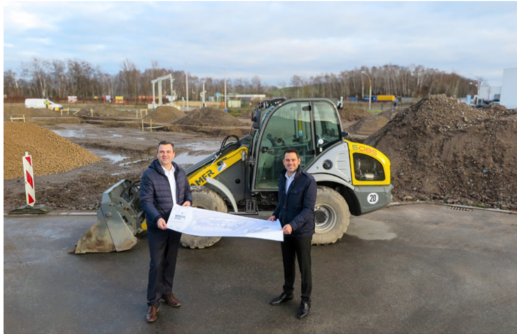
MicroStep broke ground for its new competence center, close to its existing location in Dorsten in Northern Germany (Picture: Giesers Stahlbau GmbH)
