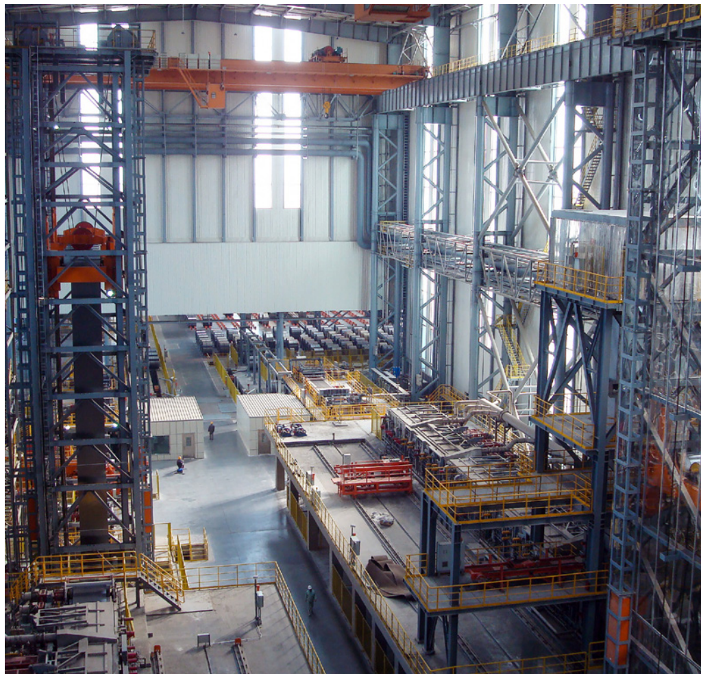
Continuous galvanizing lines CGL 5 and CGL 6 for the cold rolling mill of HBIS Tangsteel in Tangshan, Hebei Province, China (Picture: Primetals Technologies)
