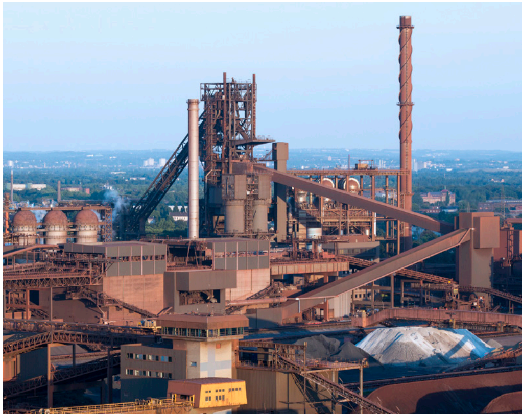
thyssenkrupp is testing the new "sequence impulse process with induced shockwaves" oxygen injection system on the Schwelgern 1 blast furnace (Picture: thyssenkrupp)
