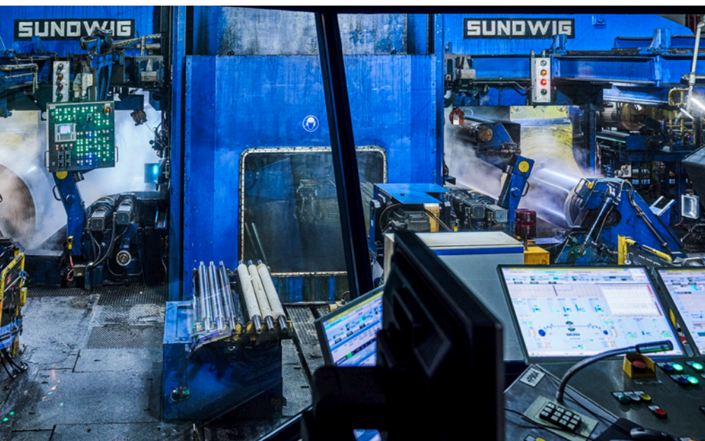
Figure 1. The "Sundwig 1350" 20-high cold rolling mill at the Dillenburg works. The VTLG can be recognised from the light blue indicator light on the mill to the right of the control panel (Picture: Wolfram Schroll / Vollmer GmbH)
