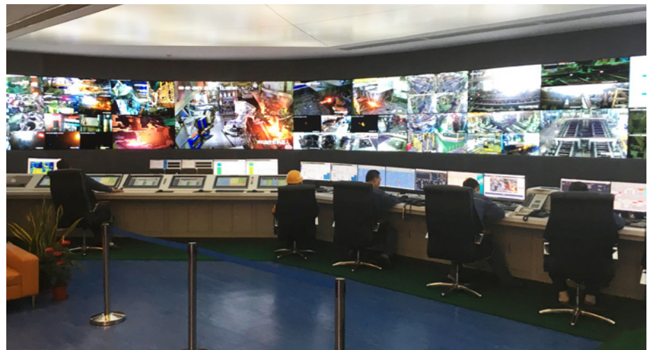
The new integrated control center of the Baosteel CC3 continuous caster at steelworks No. 1 in Shanghai increases both productivity and safety at work (Picture: Primetals Technologies)
