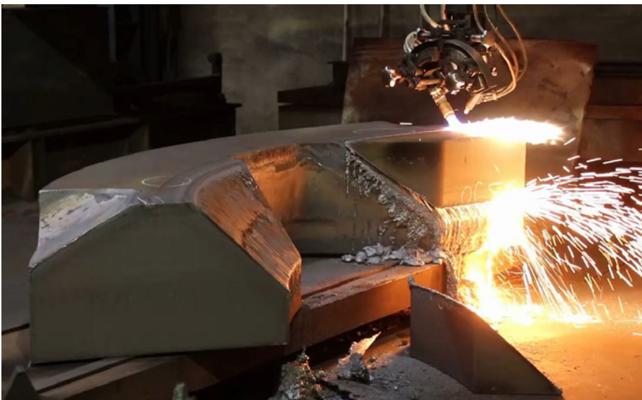
Laterally, 45-degree chamfers were cut in two levels (Picture: Jebens GmbH)
