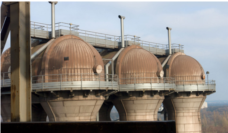
Figure 1. Pyrometers measure the temperature of the grating refractory bricks in the stove dome from the cupola (Picture: Adobe Stock / stefanbi1974)
