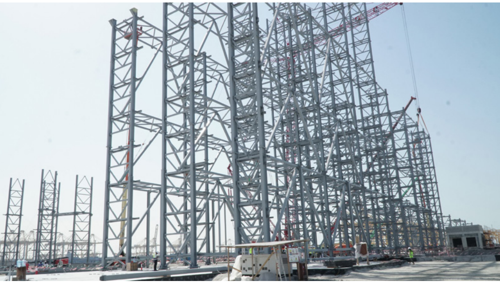
Erection of the high-bay storage (Picture: SMS group)
