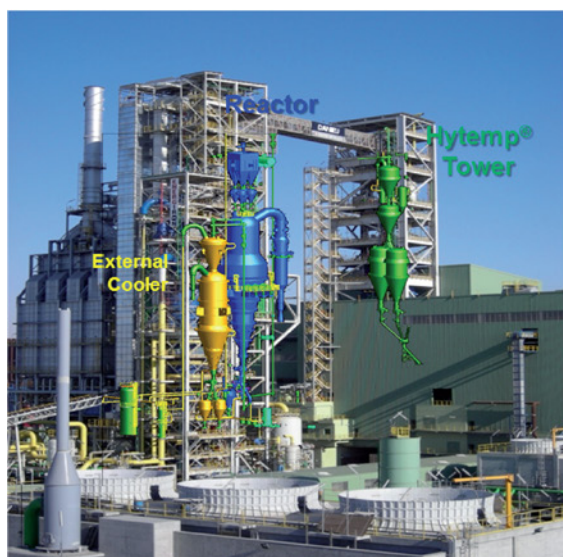
Fig. 5. The Hytemp system arrangement (left) and installation (Picture: Danieli)
