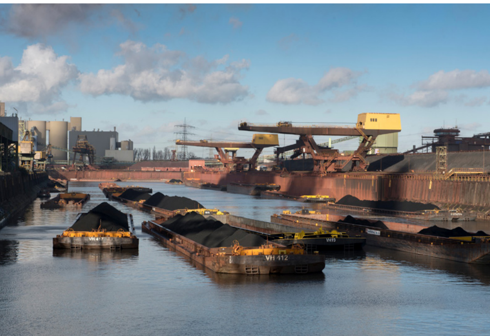
Huge amounts of raw materials are delivered to thyssenkrupp Steel's port in Duisburg every day (Picture: thyssenkrupp)
