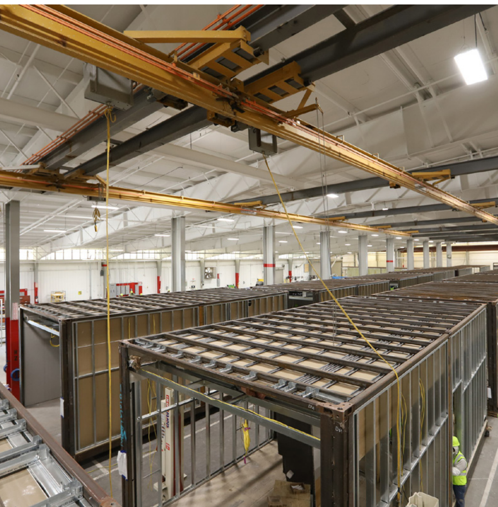
Steel-framed modules at Z Modular's Killeen facility move through the production line from fabrication to finishing before being shipped directly to the construction site
