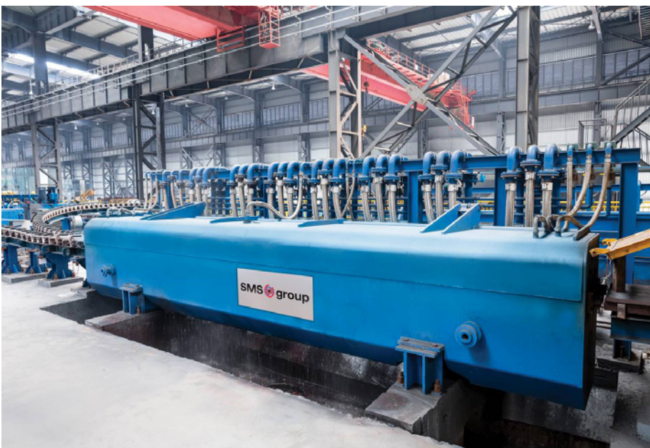
Figure 4. Intermediate cooling line with water cooling box (Picture: SMS group)
