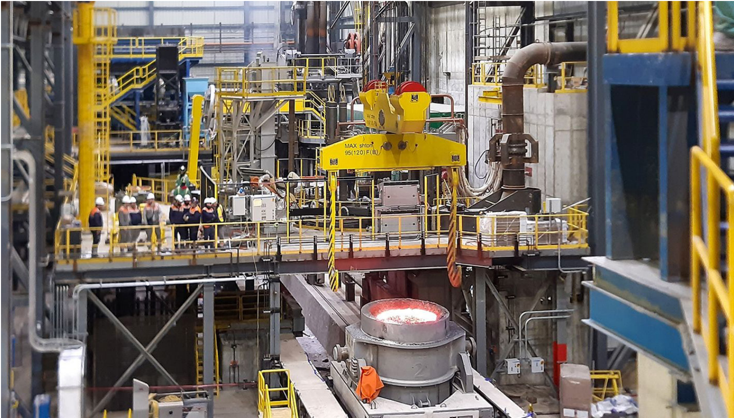
First heat at the new minimill at Nucor Steel Sedalia on January 31 (Picture: Danieli)
