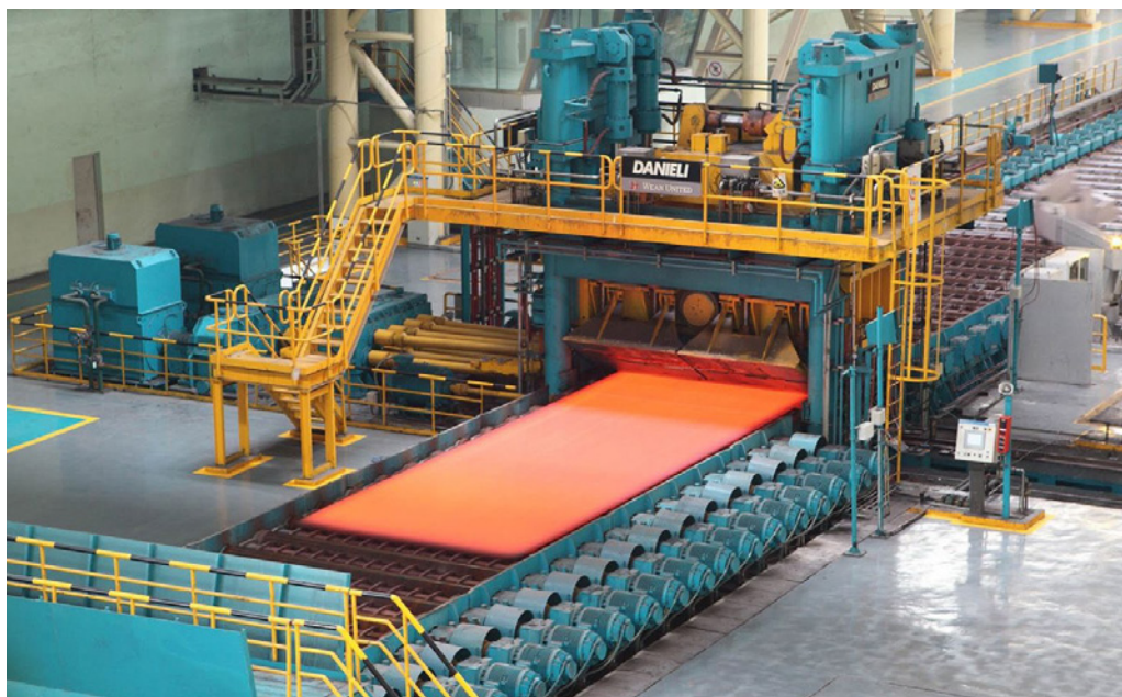
The upgrade of the wide plate mill will allow Algoma to add new grades to its portfolio (Picture: Danieli)
