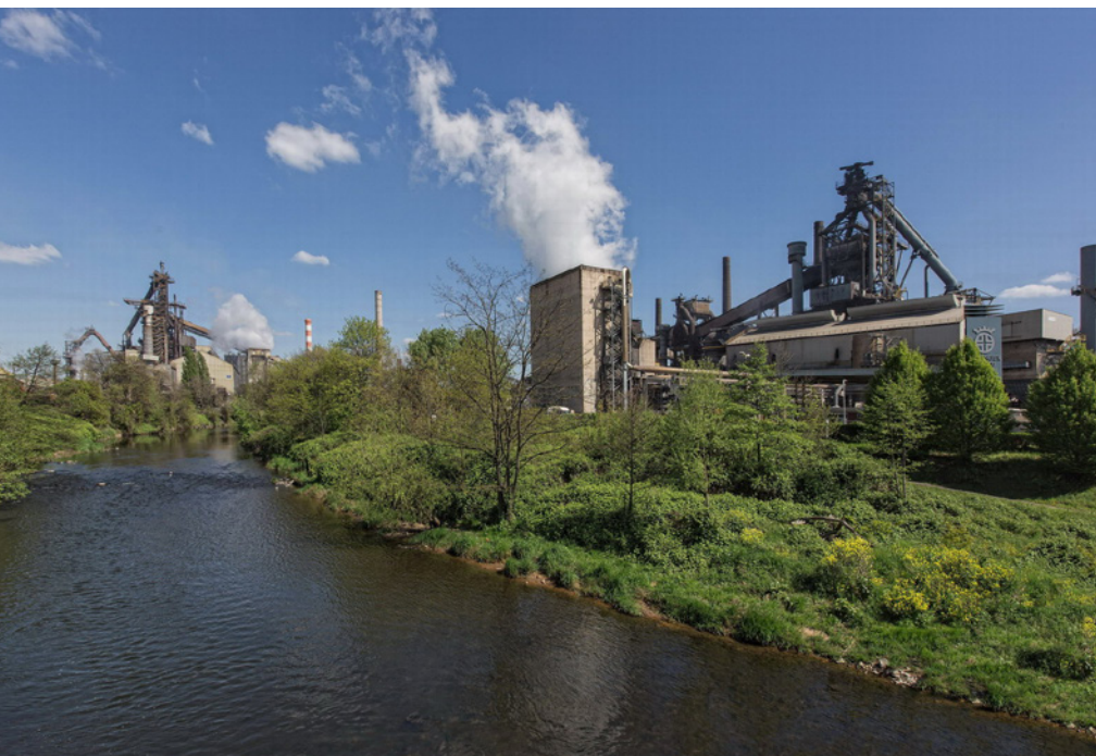
The blast furnaces of ROGESA produce hot metal to be supplied to the steel plants of Dillinger and Saarstahl (Picture: SHS)
