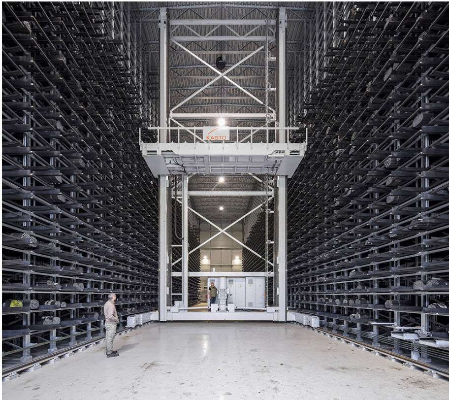
New warehouse for bright steel at Trinec Iron & Steel (Picture: Trinec Iron and Steel)
