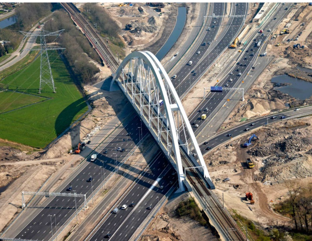
The Muiderberg railway bridge in the Netherlands (Photo: Vliegfeld Hilversum)
