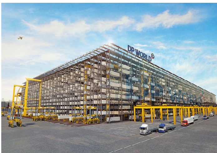
High-bay storing system for containers (Photo: SMS group)
