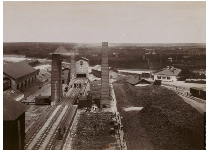
Gdantsevka ironmaking plant (1899)
